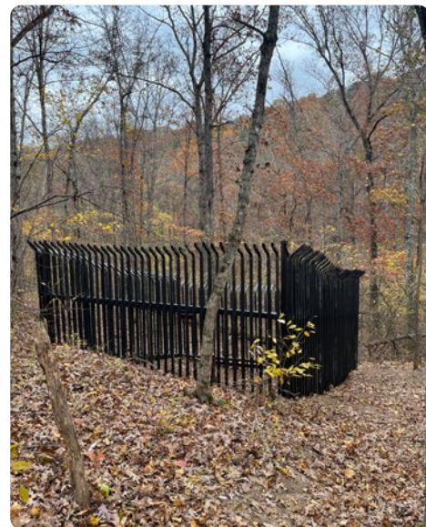
Completed Martin Cave gate.
