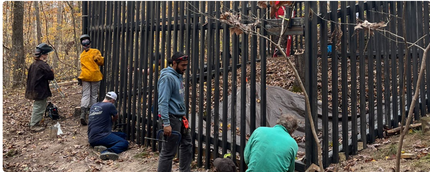
Crew members working to complete Martin Cave gate construction.
